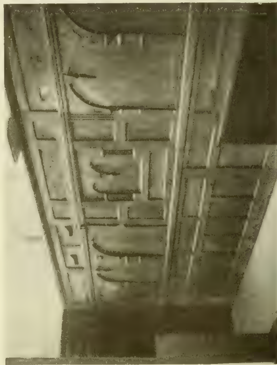
Fig. 80. ALDINGTON, KENT. Plastered woodwork of 1600-10.
